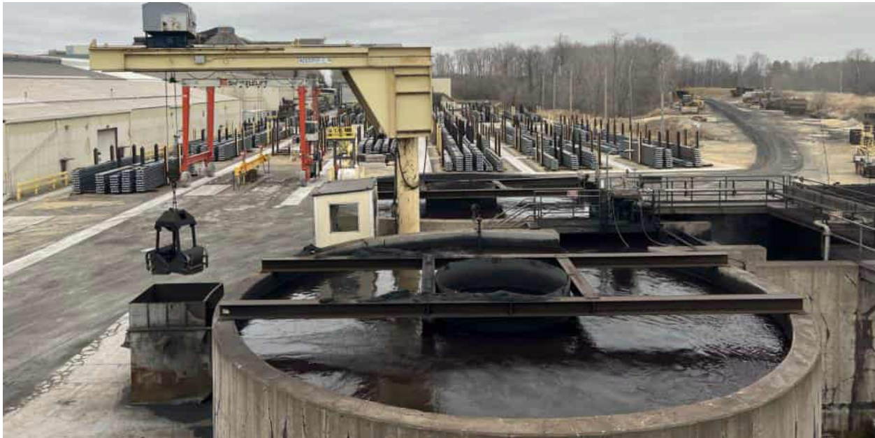
Photo #2 – Existing Scale Pits -to be Repurposed
